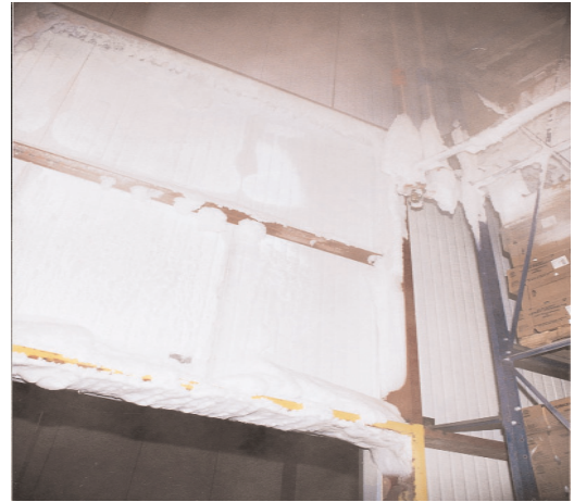
Left: Steve Cox points to a frost-free environment inside the Shaw's distribution center. Right: Before the installation of Munters equipment, frost build-up near exits formed blocks of snow and ice that threatened product quality, and forced workers to waste time chipping and thawing for hours every week.
