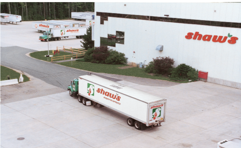
At the Shaw's frozen food distribution center in Wells, Maine, Munters desiccant units keep floors dry and save energy by reducing defrost cycles.
