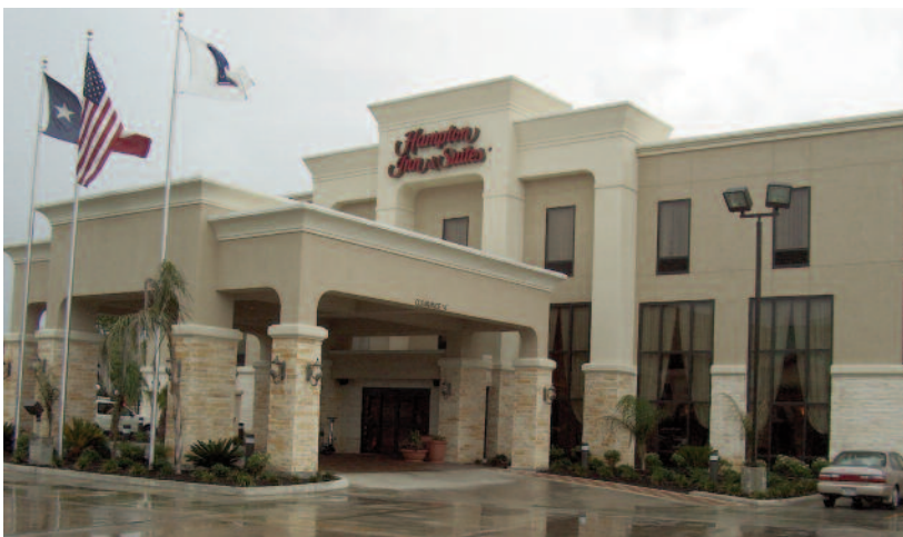
Two DryCool units were installed to treat all three floors of the Hampton Inn in Katy, Texas.
