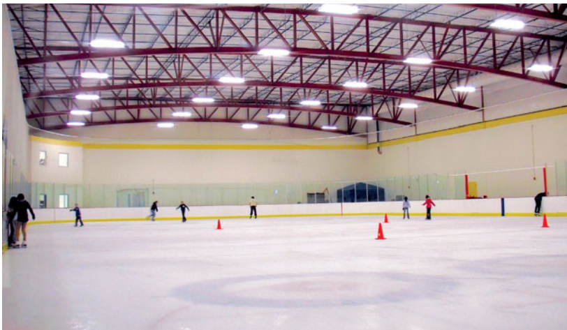
The Chaparral Ice rink in Austin, TX was the first rink to install the all new Munters FreeDry™ system over a year ago. The rink realized substantial energy savings with the more energy efficient technology.
