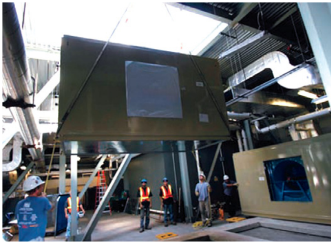
Directly Above: The dehumidification system had to be hoisted on to the roof of the ACC by crane in three pieces. Right: One of the two units installed. Top Left: Low-level fog obscures the ice action and leads to safety problems.
