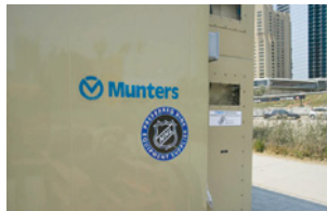
Directly Above: The dehumidification system had to be hoisted on to the roof of the ACC by crane in three pieces. Right: One of the two units installed. Top Left: Low-level fog obscures the ice action and leads to safety problems.
